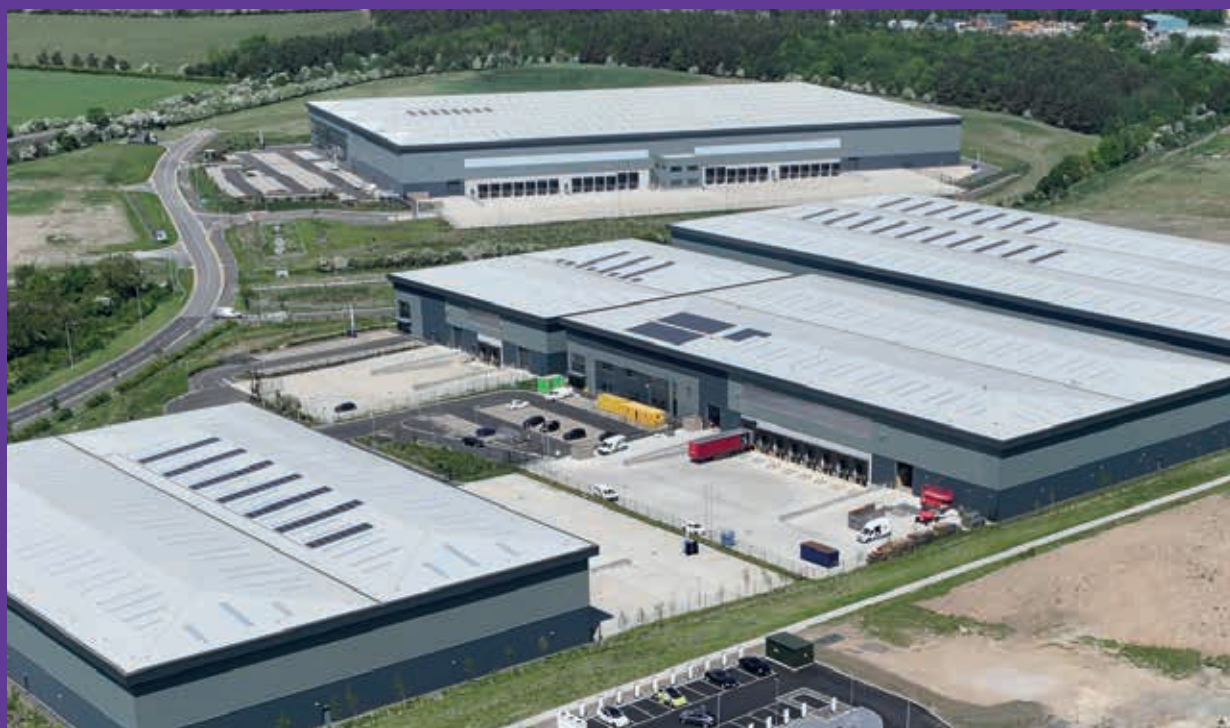
EXISTING INDUSTRIAL UNITS AT INTEGRA 61
